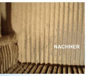
Boiler tubes after sufficient sootblowing
